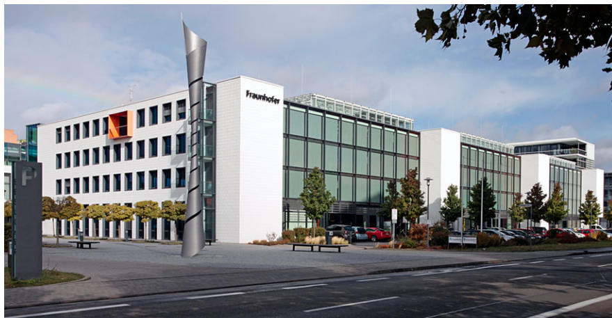
Fig. 3 Institute building of the ITWM at the Fraunhofer Center in Kaiserslautern (Photo: G. Ermel, Fraunhofer ITWM)
