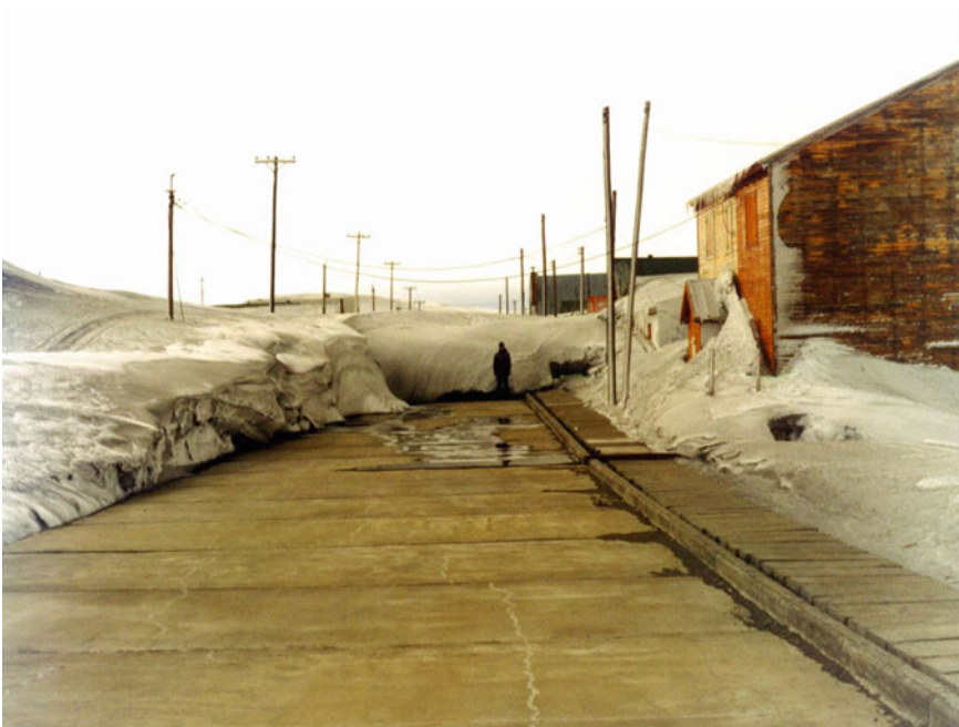
Fig. 11.9 Ice and snow from the streets of Copahue are removed by a geothermal heating system
