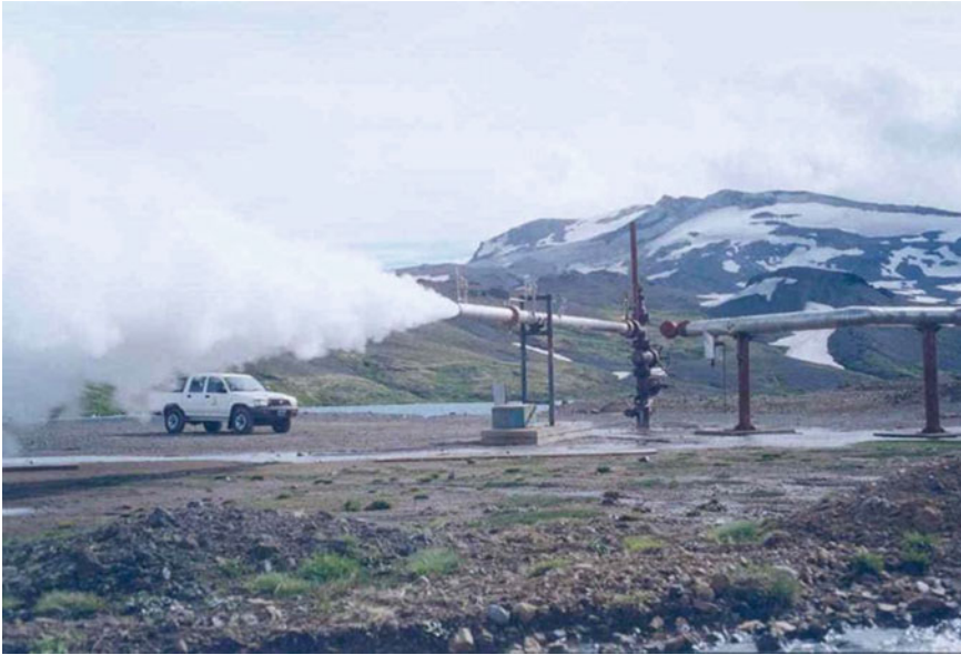
Fig. 11.8 The COP-4 well and the steam pipeline
