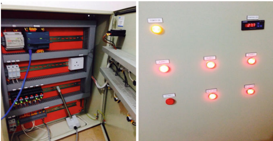
Fig. 3 Our built Siemens PLC S7-1200 temperature sensor
