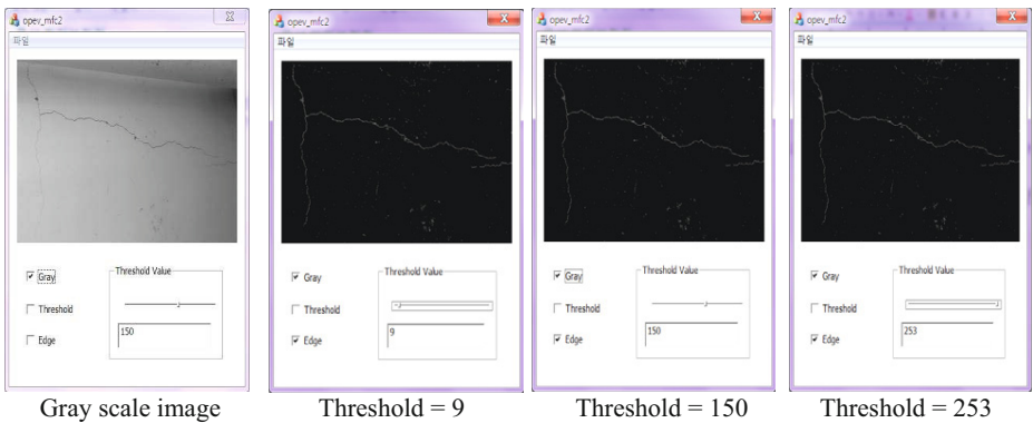
Fig. 5. Experiment of Detecting the Crack of Buildings
