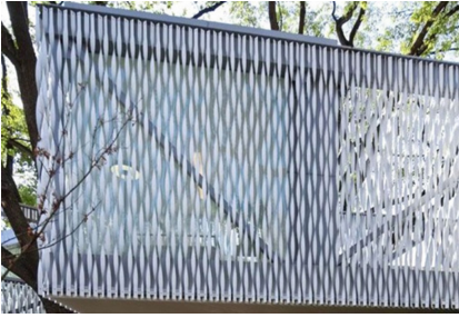
Fig. 12. Element’s distortion: twisted elements: huaxin business center, in Xuhui, China.
