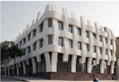
Fig. 14. Element’s distortion: interlaced elements - argul weave building, in Bursa, Turkey.
