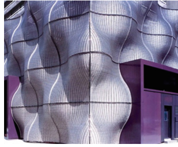
Fig. 5. Facade geometry: sinusoidal and co-sinusoidal facade - boiler house at Guy's Hospital, in London, UK.
