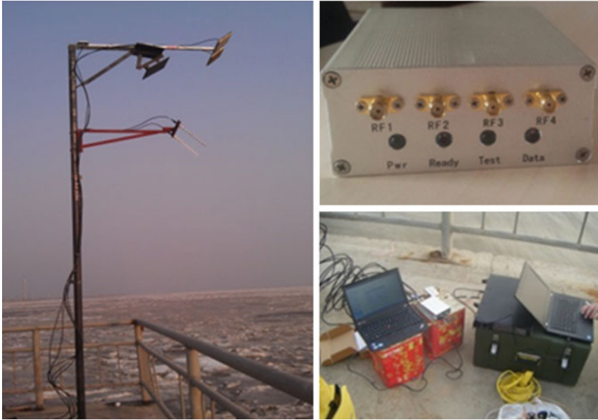
Fig. 24.1 Equipment and GNSS receiving data
