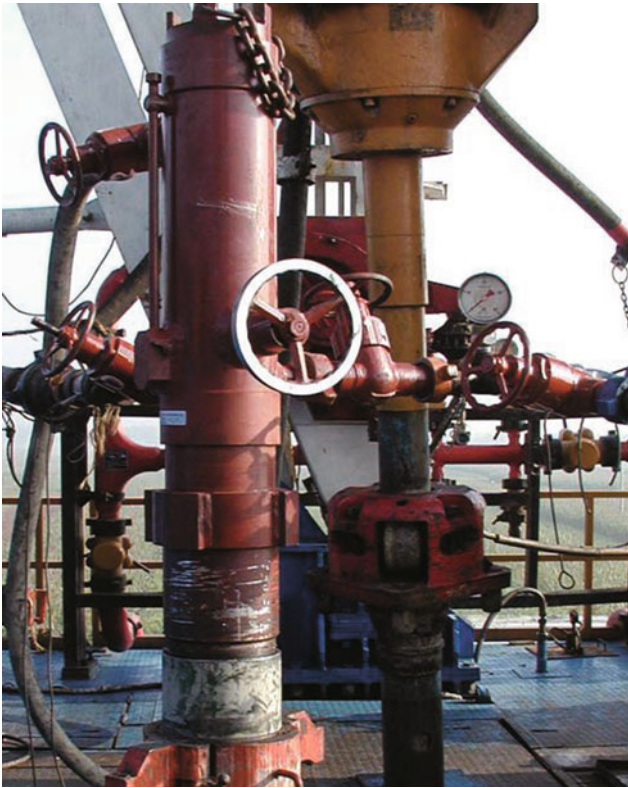
Fig. 10.15 Cement head for 273.0 mm intermediate casing cementation
