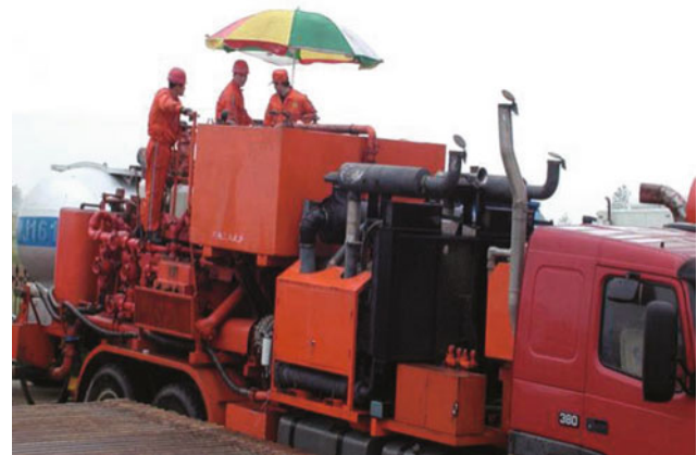
Fig. 10.19 Operation of 193.7 mm casing cementation
