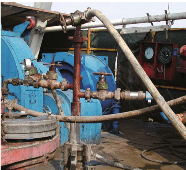
Fig. 10.24 Cement head for 127 mm tail pipe cementation
