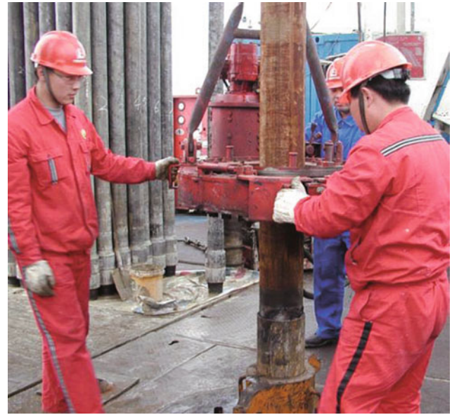
Fig. 10.18 Running 193.7 mm casing
