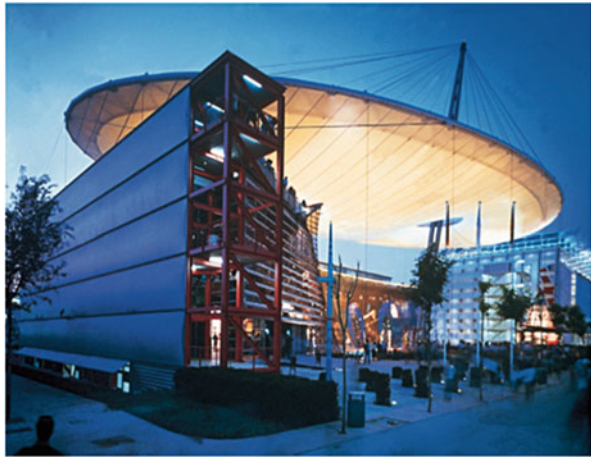
Fig. 16.41 Suspended construction ( Source: Ceno Tec GmbH )
