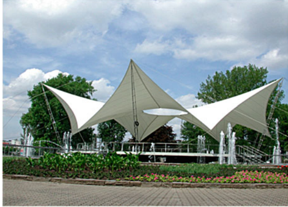
Fig. 16.40 Mechanically tensioned structure ( Source: Ceno Tec GmbH )
