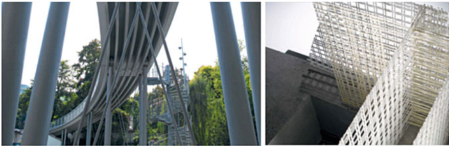
Fig. 16.33 Pedestrian bridge in Albstadt, Germany (Source: Groz-Beckert KG)
