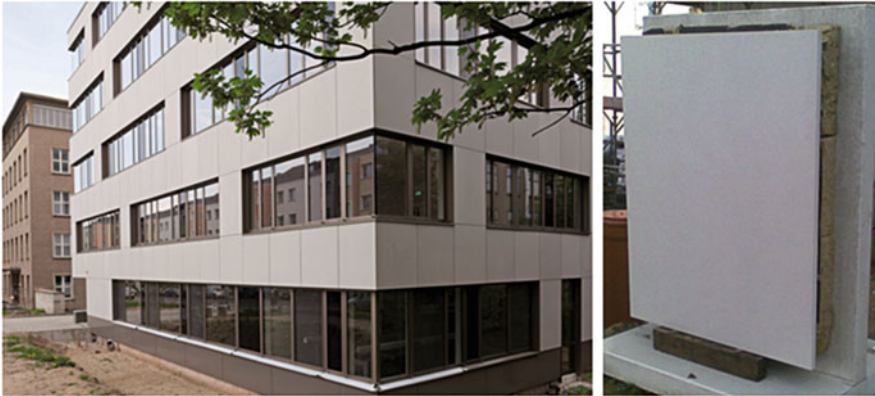
Fig. 16.31 betoShell ® textile concrete facade elements ( Source: Ulrich van Stipriaan)
