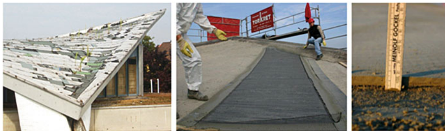
Fig. 16.29 Reinforcement of the hyper shell structure at FH Schweinfurt
