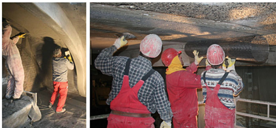
Fig. 16.30 Installation of the textile concrete reinforcement layer
