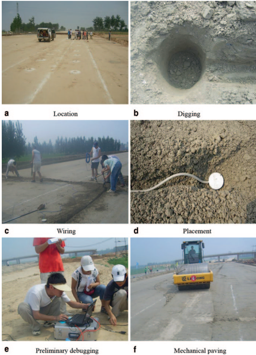
Fig. 10.4 Sensor layout process. a Location. b Digging. c Wiring. d Placement. e Preliminary debugging. f Mechanical paving
