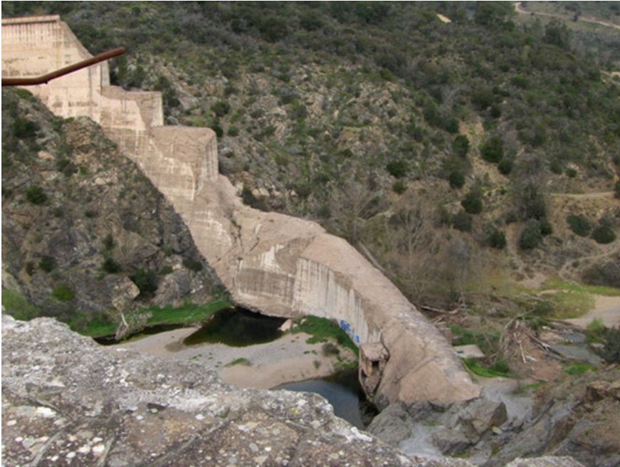
Fig. 7.2 Failure of the Malpasset Dam (France) in 1959 (photo Irstea)
