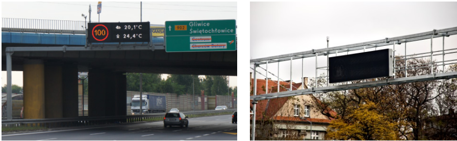
Fig. 1. The VMS signs and the weather stations in Chorzów [own study]
