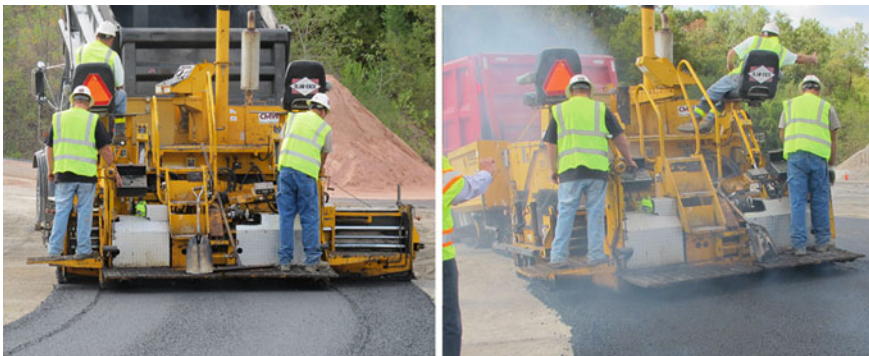
Fig. 10.2 Paving of WMA (left) using foaming technology and HMA (right)
