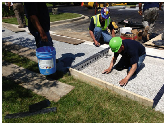
Fig. 8.8 Installation of precast hollow core pervious concrete pavement panels
