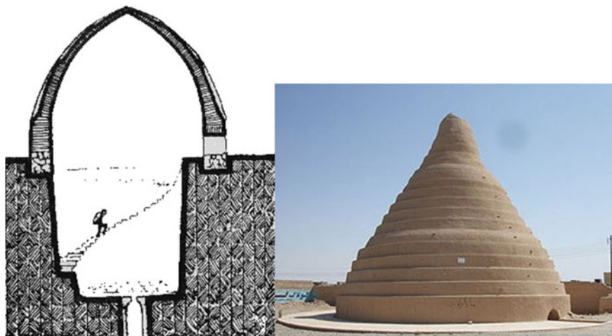
Fig. 18.15 A yakhchal (ice house) in ancient Persia, a place to store ice in summer
