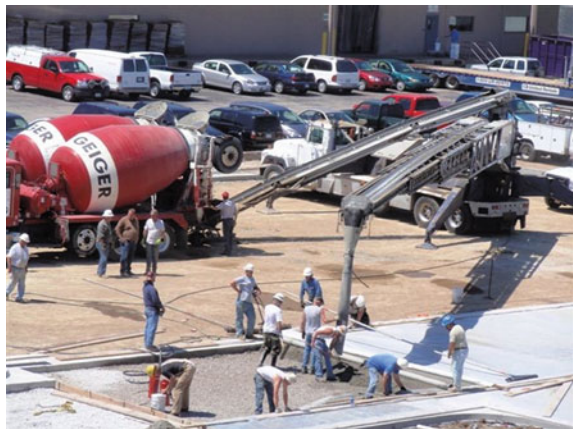
Fig. 8.5 Pervious concrete construction using a belt placer
