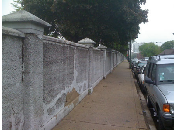
Fig. 8.9 Reinforced pervious concrete walls
