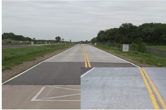
Fig. 8.7 Pervious concrete overlay for noise reduction
