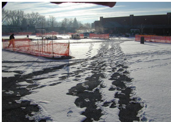
Fig. 8.6 Reduced slip and fall potential of snow-covered pervious concrete
