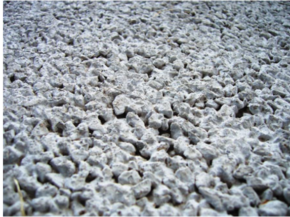
Fig. 8.4 Pervious concrete surface texture
