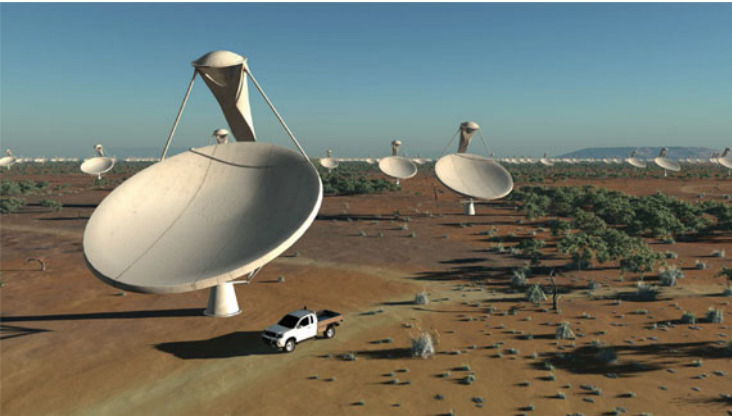
Fig. 1.7 SKA parabolic dishes for medium frequencies of about 350 MHz–14 GHz. Graphics: Swinburne Astronomy Productions and SPO
