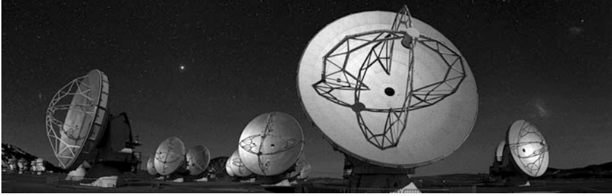
Fig. 2.1 Several ALMA antennas at the Chajnantor plateau. The 12-m diameter ALMA antennas are seen in the foreground, while in the far left a cluster of smaller 7-m antennas for the ACA are also visible. (Photograph credit: Babak Tafreshi)
