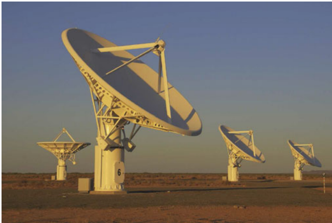
Fig. 1.10 Antennas of the KAT-7 array (photo: Maik Wolleben, SKA Project South Africa)
