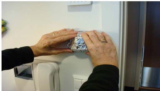
Fig. 3. A light sensor ‘hacked’ with foil. Photo: Finken
