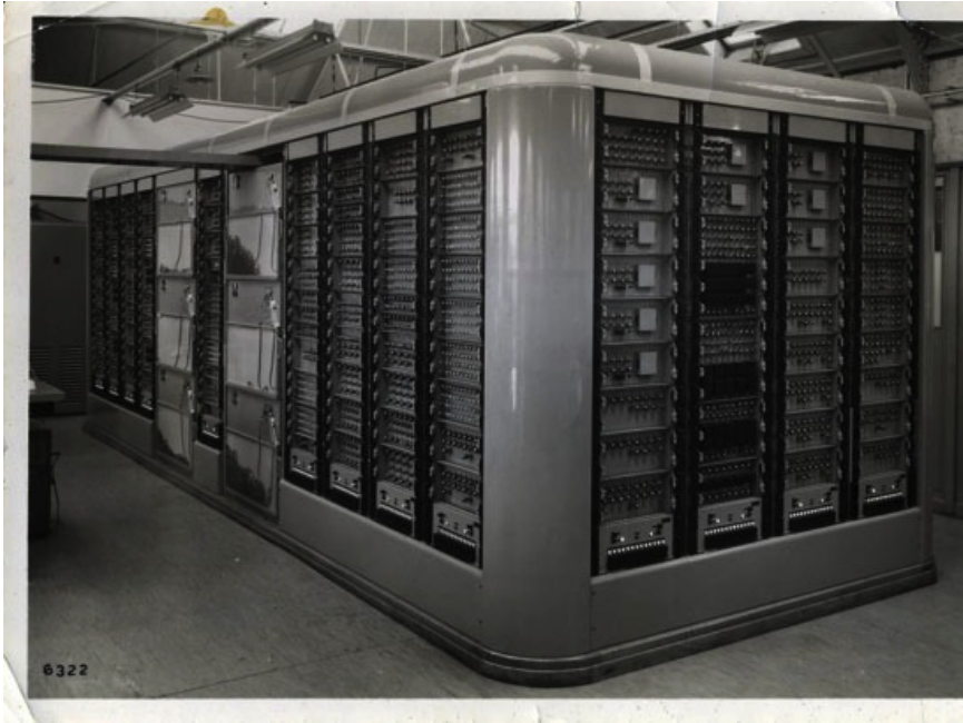
Fig. 5. The “initial” MMIF (with 17 racks), front view (Source: [19], photo I)
