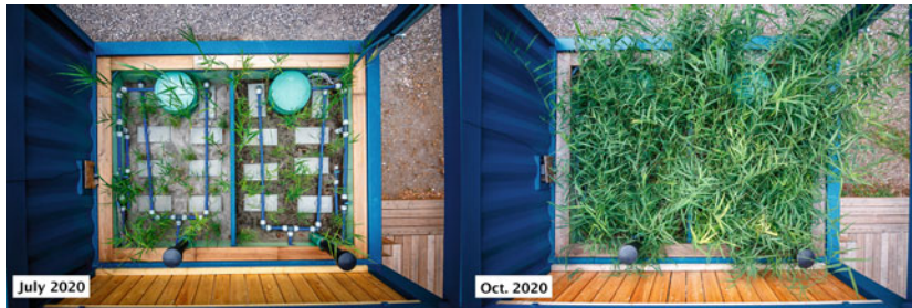
Fig. 7.2 Constructed wetland at the beginning of infiltration with light greywater (left) and after three months (right). (Photos: J. Rettig)
