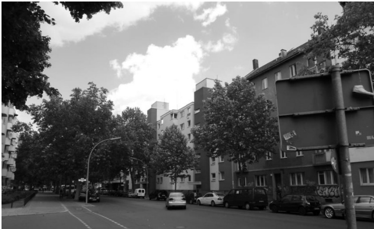
Figure 1b: Kreuzberg Ost. View of Gründerzeit buildings on Görlitzer Straße (Görlitzer Park on the right) (image: Christine Stegner)
