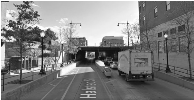
Fig. 7 Railroad Viaduct, Halsted and Sixteenth Street, looking north on Halsted Street (above). The railroad tracks are now located on the viaduct that crosses over Halsted Street. Google Maps Street View (retrieved May 2016).
