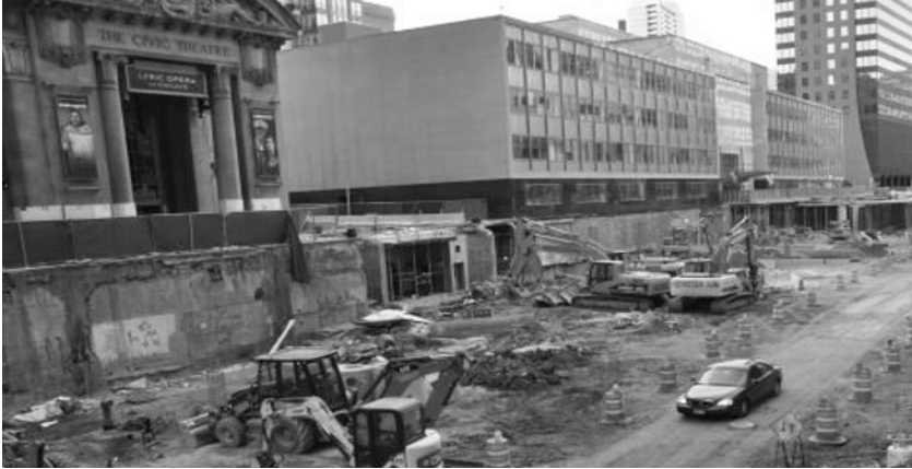
Fig. 1 The original Market Square area, looking south on Market Street during (re)construction of the two-level Wacker Street Drive. Market Street would correspond to what is now Lower Wacker Street Drive.
