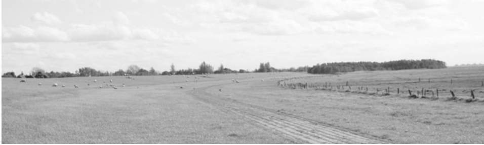
Fig. 5.7 The shape of a main dike in Lower Saxony, northern Germany. The photograph shows the sea side of the main dike with a gentle slope and a salt marsh in front of the dike. ©Frank Ahlhorn
