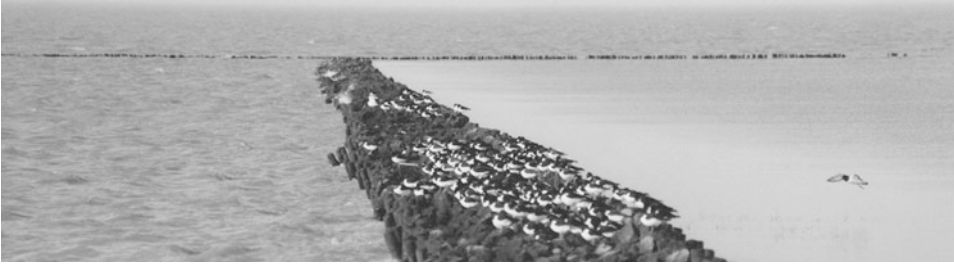
Fig. 6.6 Brush wood groynes reducing wave impacts and, though enhancing sedimentation in order to enable mud flats to grow with sea level rise (subsequently reducing risk at flooding). ©Frank Ahlhorn
