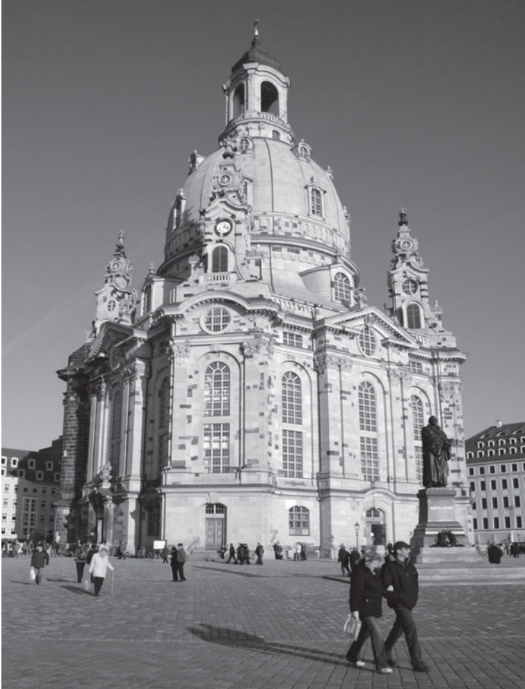
Figure 1: Rebuilt Church of Our Lady in Dresden, Germany: The remaining parts of the original are visible as dark spots within the new structure. (Author 2006)
