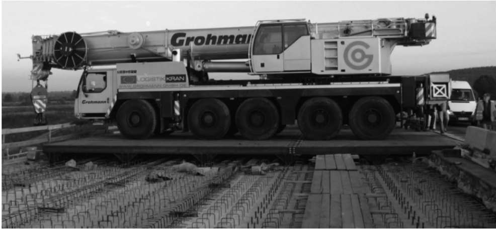
Figure 38: Crane on temporary platform.
