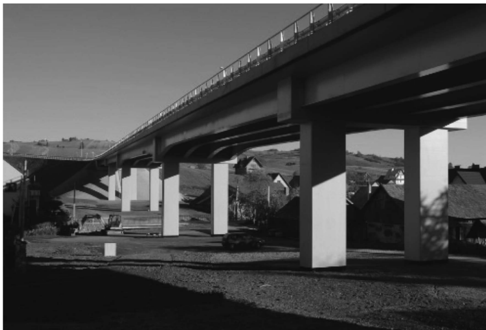
Figure 25: General bottom view of the bridge in Kluszkowce
