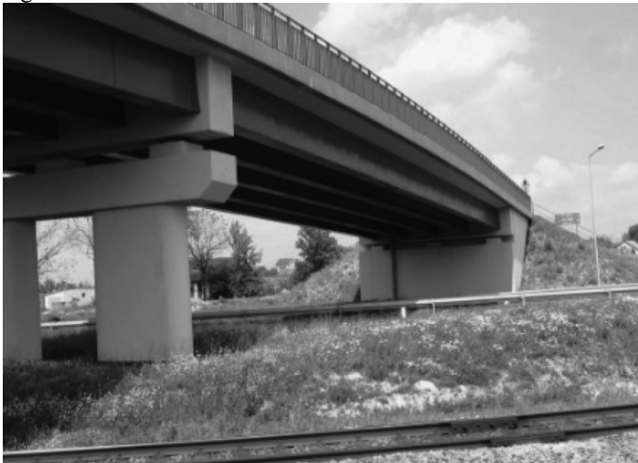
Figure 1: Two-span continuous beam (43m+43m) VFT viaduct next to Kije
