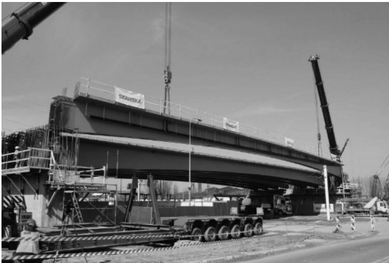
Figure 10: Placement of prefabricated girder of 63 m frame on Route Sucharskiego
