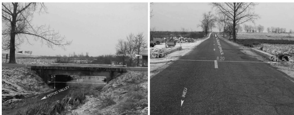
Figure 2: General view of the bridge and access ramps
