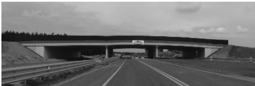
Figure 27: General view of crossing for animals PE1
