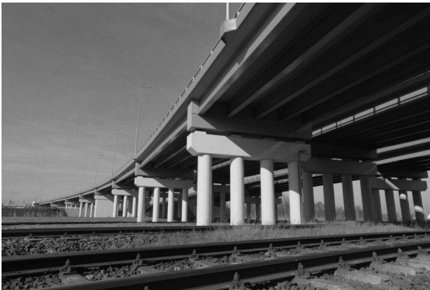
Figure 34: View of the decks of realized viaducts WD7 and WD8, Gdańsk, Poland
