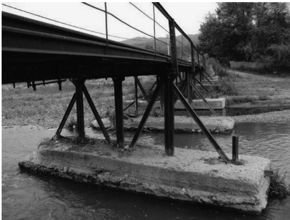
Figure 1: Existing bridge over the Bistrița River at Frânceşti
