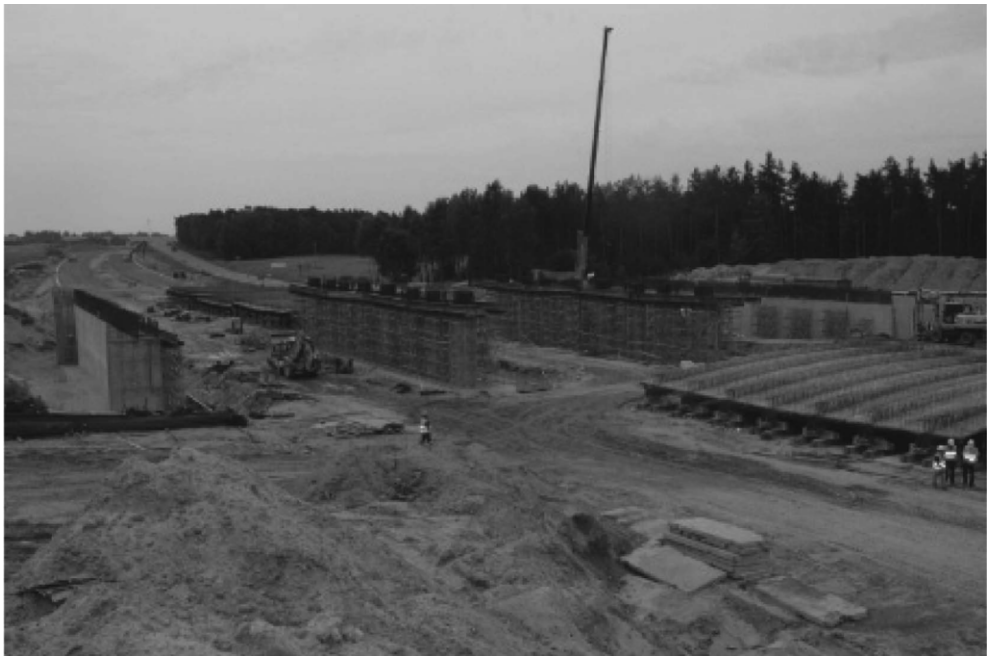
Figure 34: General view of construction site when full prefabrication used
