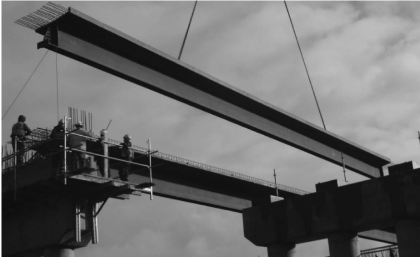
Figure 32: Setting of prefabricated beam at WD8
