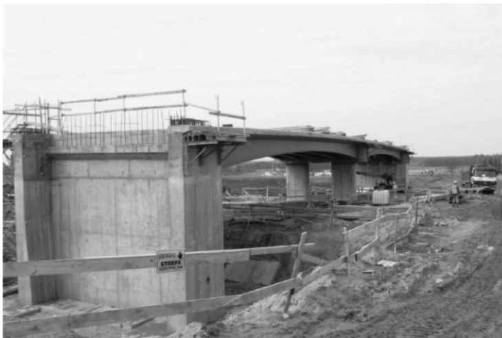
Figure 19: 19 VFT frame without finishing works and embankments
