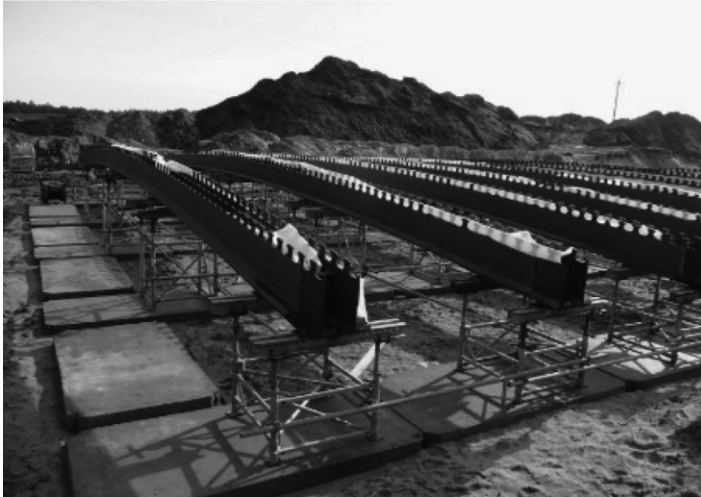
Figure 29: Steel shapes at prefabrication stand
