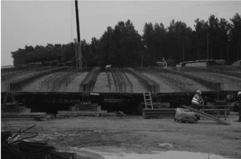
Figure 33: Large width of prefabricated girders for fan-shaped span
