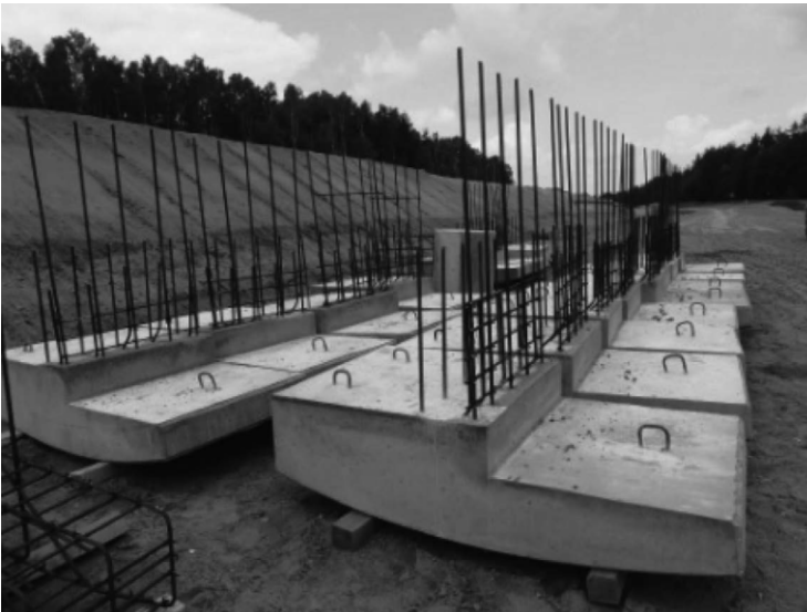
Figure 25: Prefabricated elements of cornice
