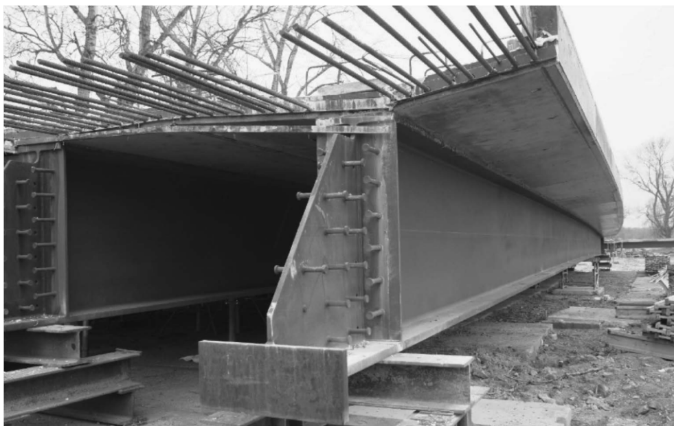
Figure 31: VFT prefabricates for WD8
