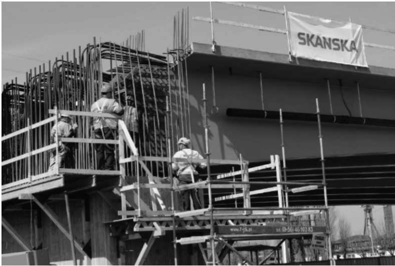
Figure 11: Construction of frame corner of 63 m frame on Route Sucharskiego
