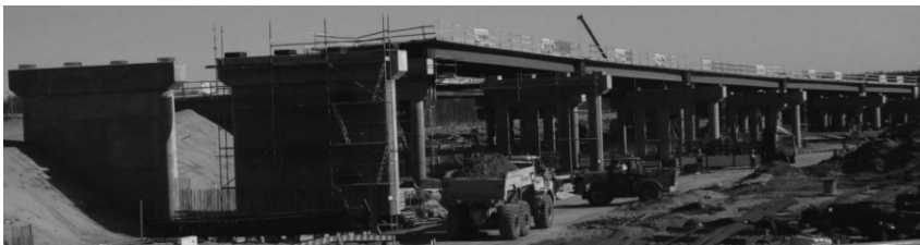
Figure 33: WD8 construction site
