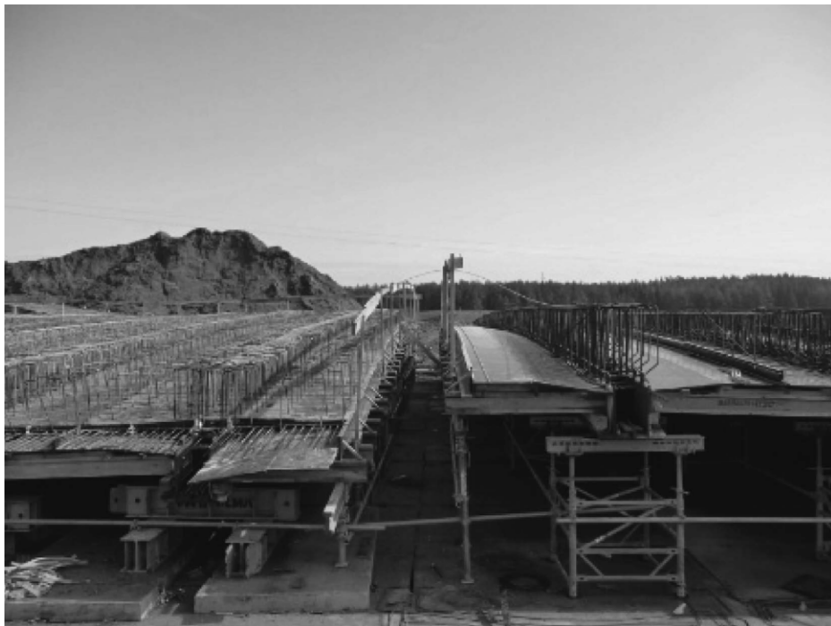
Figure 31: Reinforcement (at right) and realized (at left) prefabricated VFT-WIB girders
