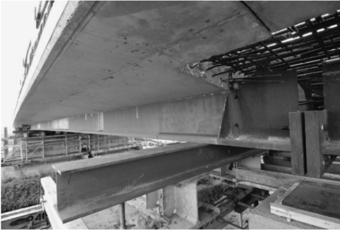
Figure 5: Prefabricated girder on temporary supports
