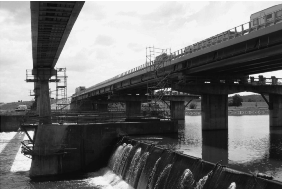
Figure 43: Realized first line of VFT continuous beam (from right)
