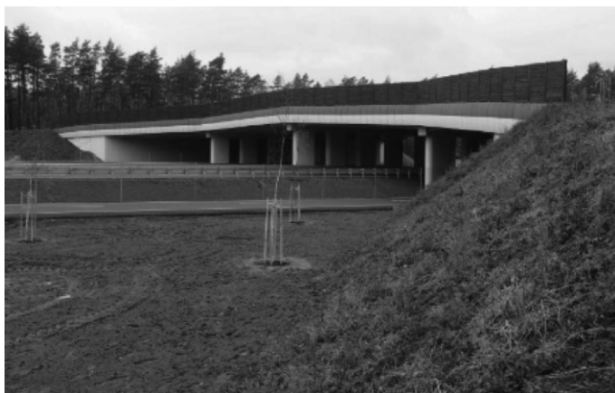
Figure 26: General view of crossing for animals PE4
