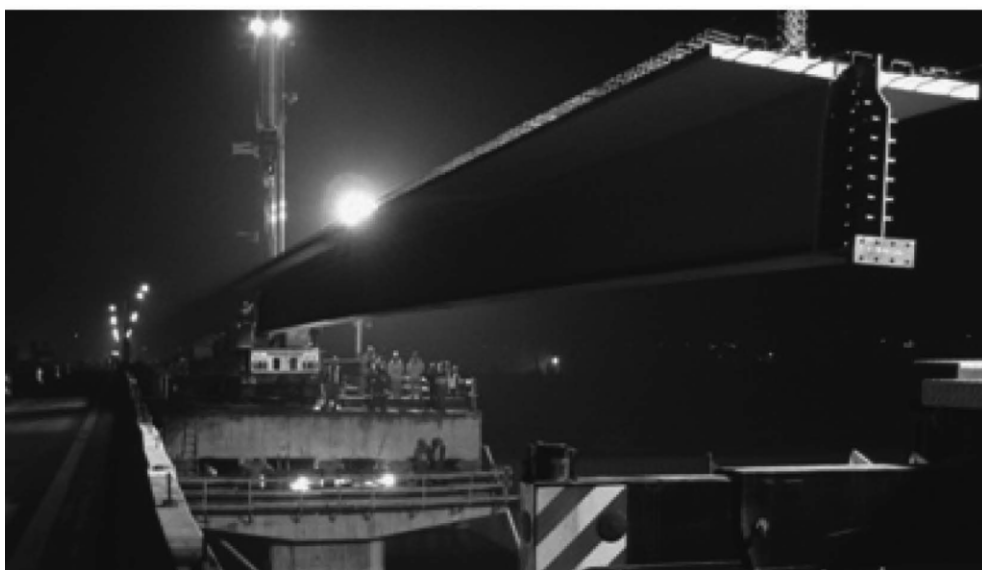
Figure 44: Montage of prefabricated elements
