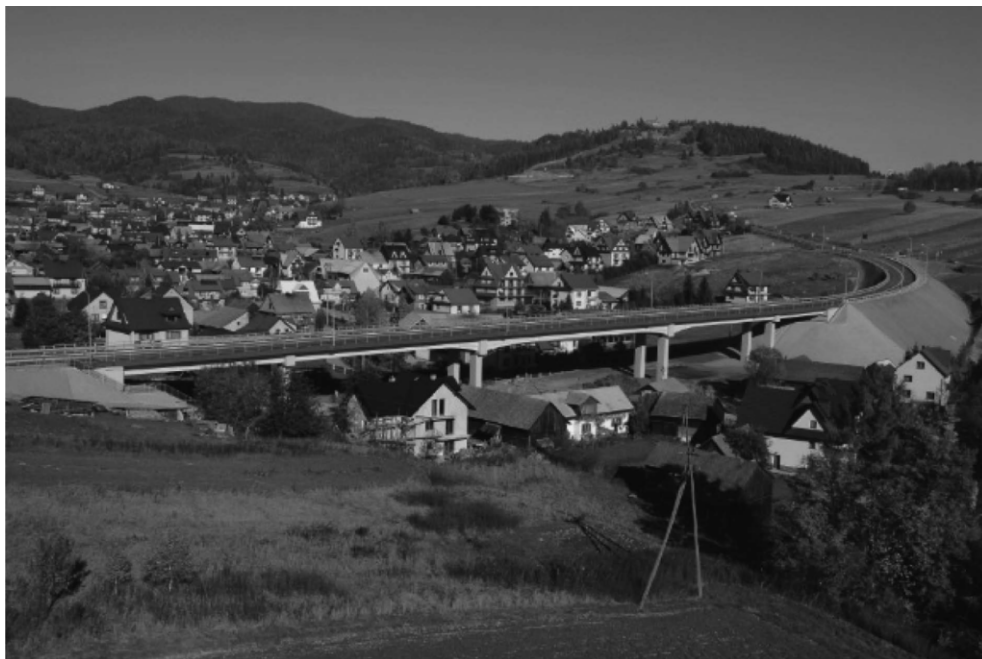
Figure 21: General view of the bridge in Kluszkowce
