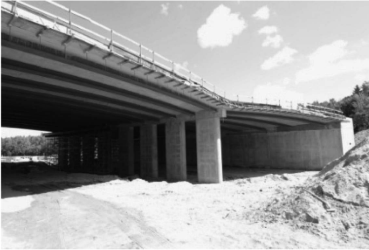
Figure 24: PE4 structure before construction of embankments
