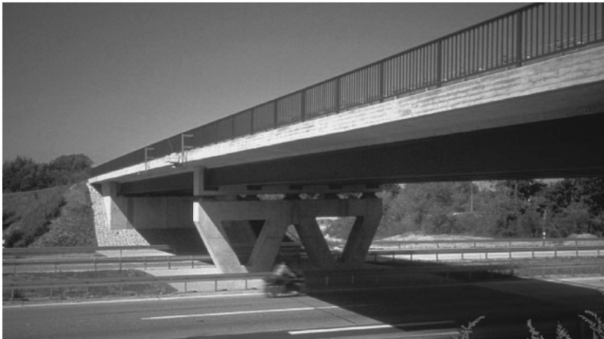
Figure 2: Composite bridge over A5 highway at Bremgarten (D) with 2 x 30m span, rolled beams in HISTAR460 and concrete crossbeams
