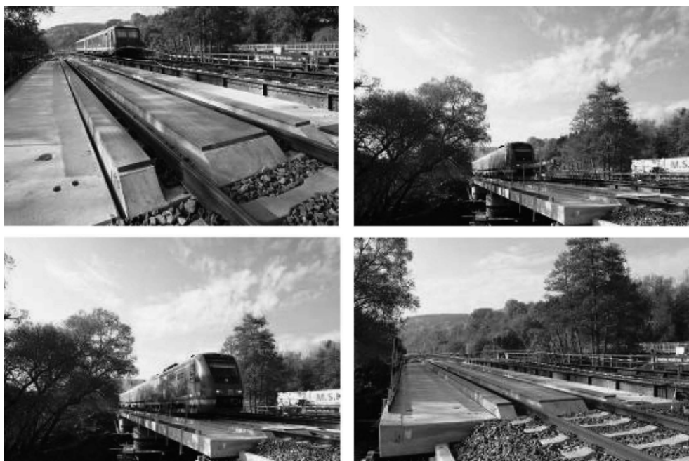
Figure 3: Simmerbach bridge – General view
