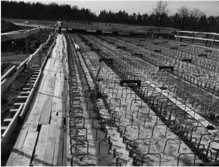
Figure 18: Upper surface of prefabricated VFT girders
