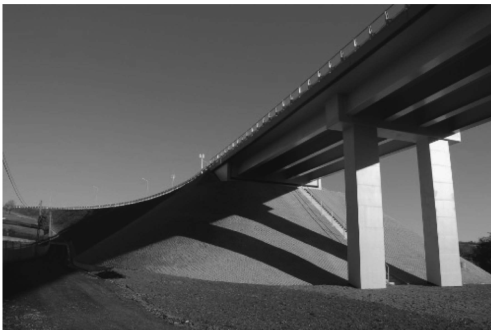
Figure 26: Abutment and first pillar of the bridge in Kluszkowce
