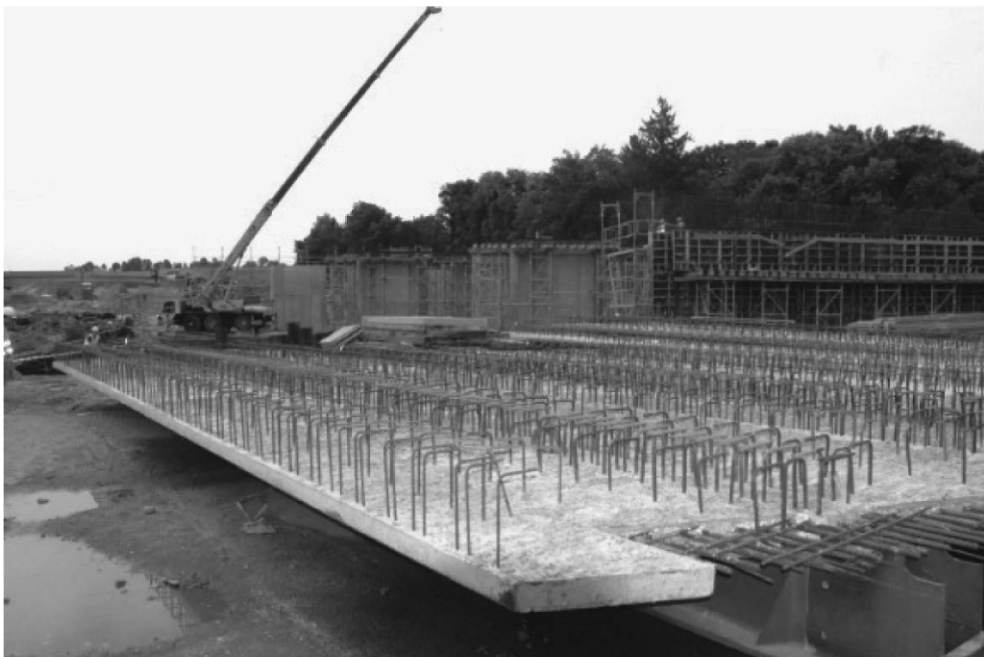
Figure 4: Prefabricated girder of road bridge on site
