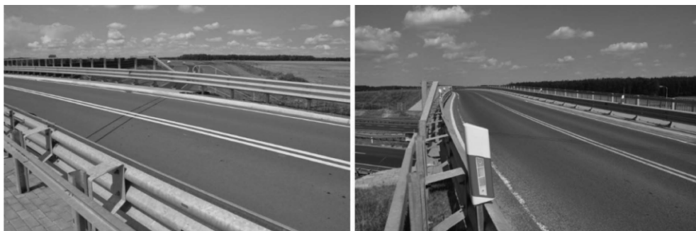
Figure 20: Asphalt layer at the abutment region (different skews)
