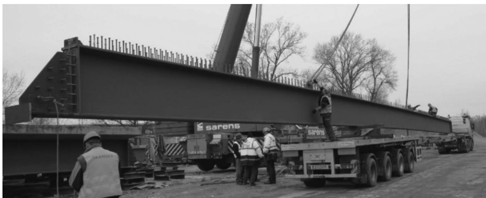
Figure 30: Steel beam for WD8 girders
