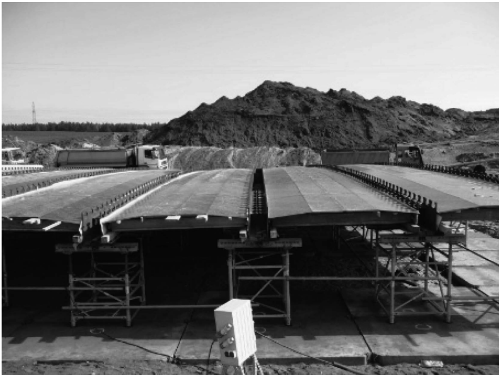
Figure 30: Scaffolding of prefabricated VFT-WIB girders
