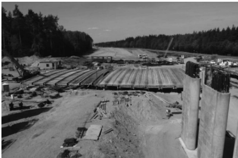
Figure 19: Prefabrication of girders for second line of PE4 structure
