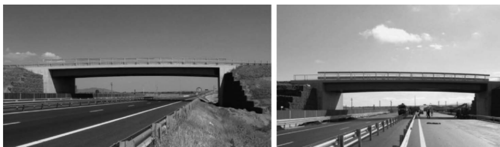
Figure 6: Integral overpasses over the A1 Motorway, section Orastie – Sibiu
