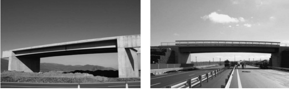
Figure 8: The final structure and its equipment.
