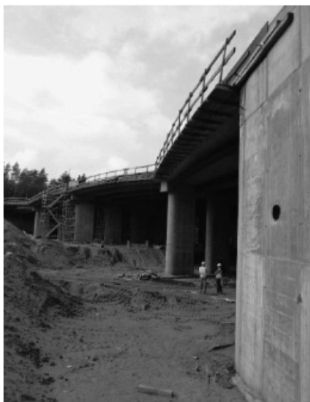
Figure 23: PE4 structure before construction of embankments
