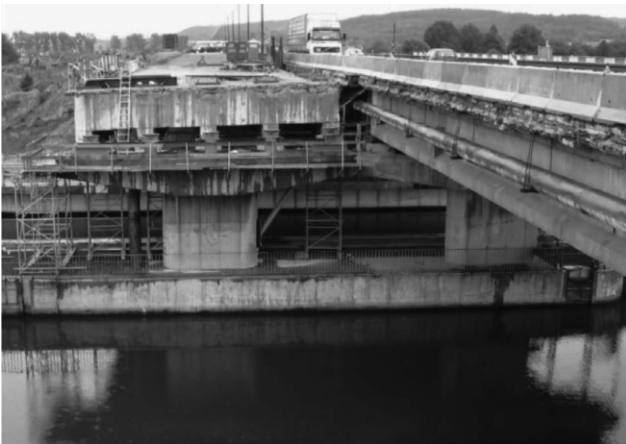
Figure 37: Old concrete span removed at the bridge at highway A4 km 417+888
