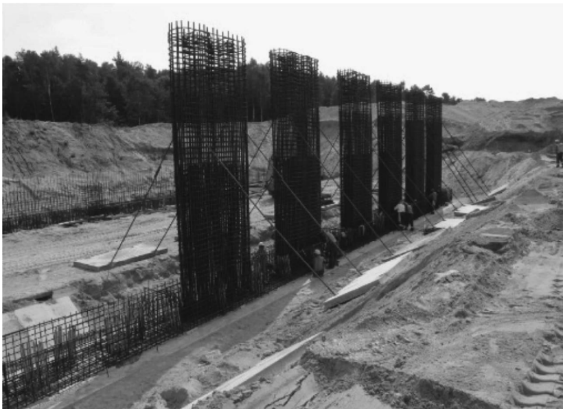
Figure 14: Reinforcement cages of pillars
