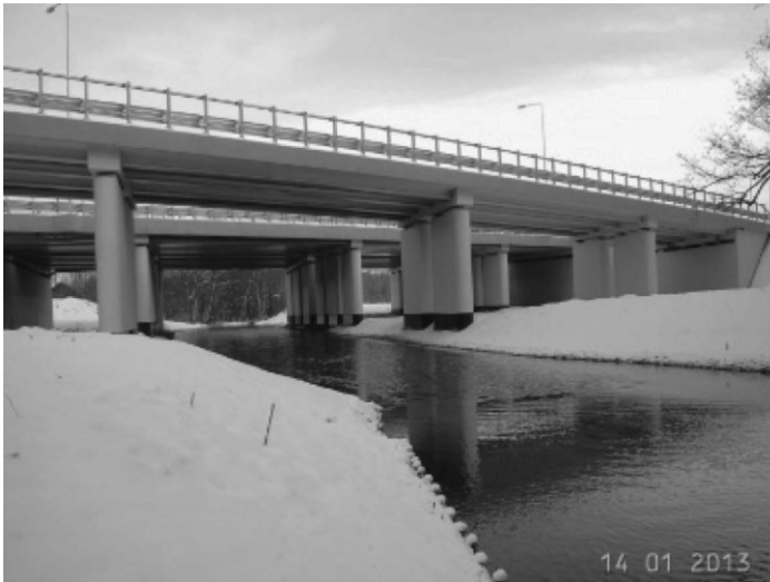
Figure 6: Bridges MD1 and MD2 [picture from: http://s7.olsztynek-nidzica.zaprojektuj-zbuduj.pl/roboty-mostowe.html ]
