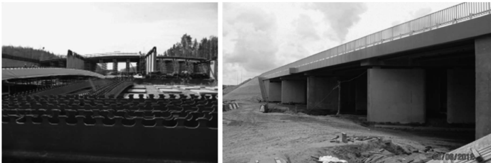
Figure 4: PE4 bridge in Poland – PreCoBeam technology
