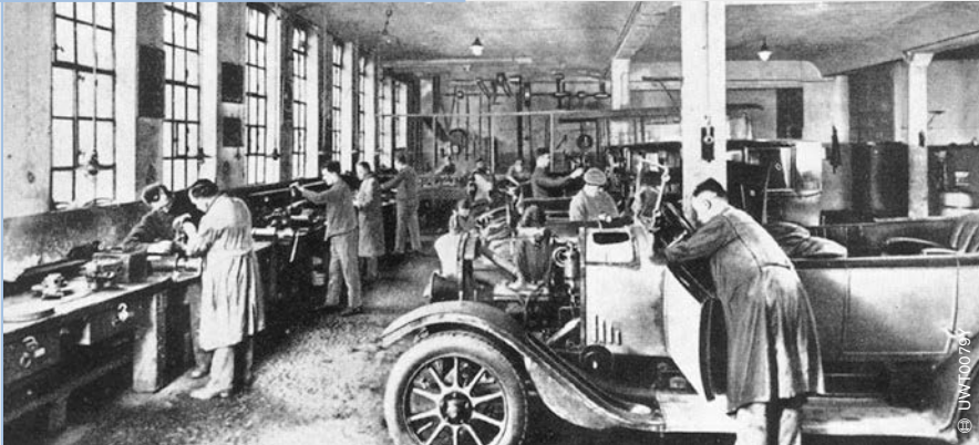
1 A repair operation in the year 1925 (Photo: Bosch)
