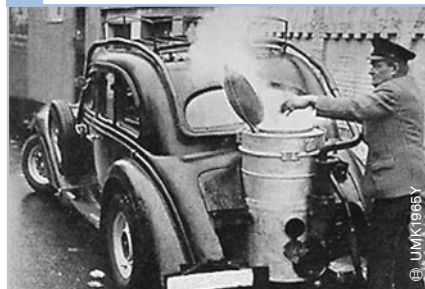
22 Wood-gas generator system on a 1936 Adler Diplomat
