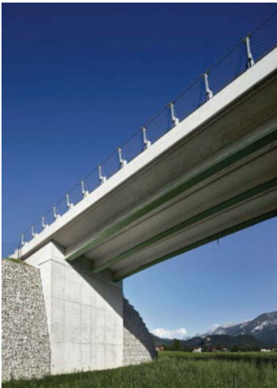
Figure 23: Bottom view on the VFT-WIB girders at Kuchl bridge (A)
