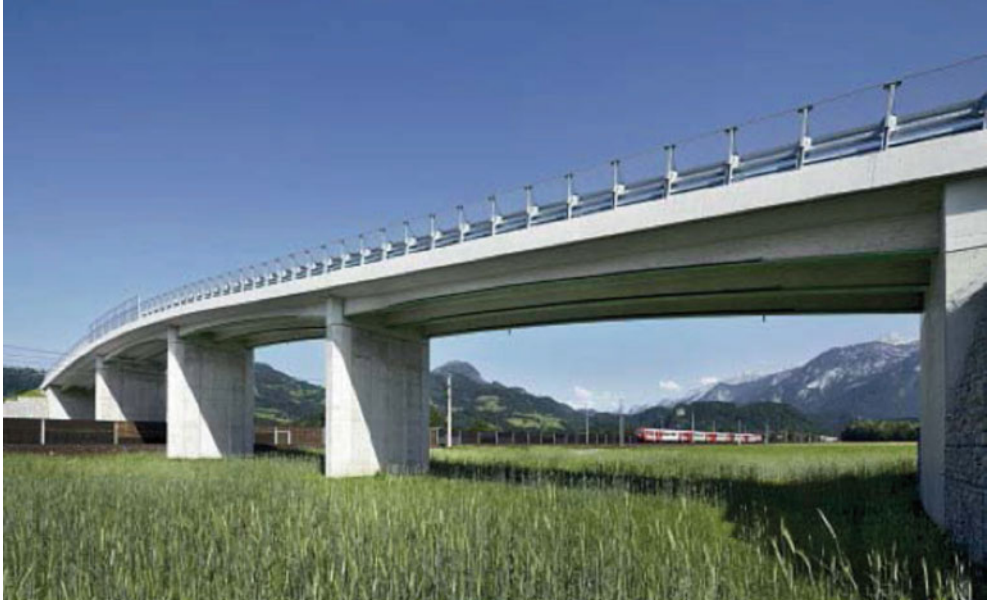
Figure 22: View on Kuchl viaduct (A)
