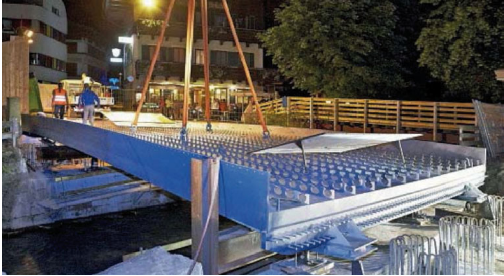
Figure 37: Placing of the steel multi-box girder at the construction site
