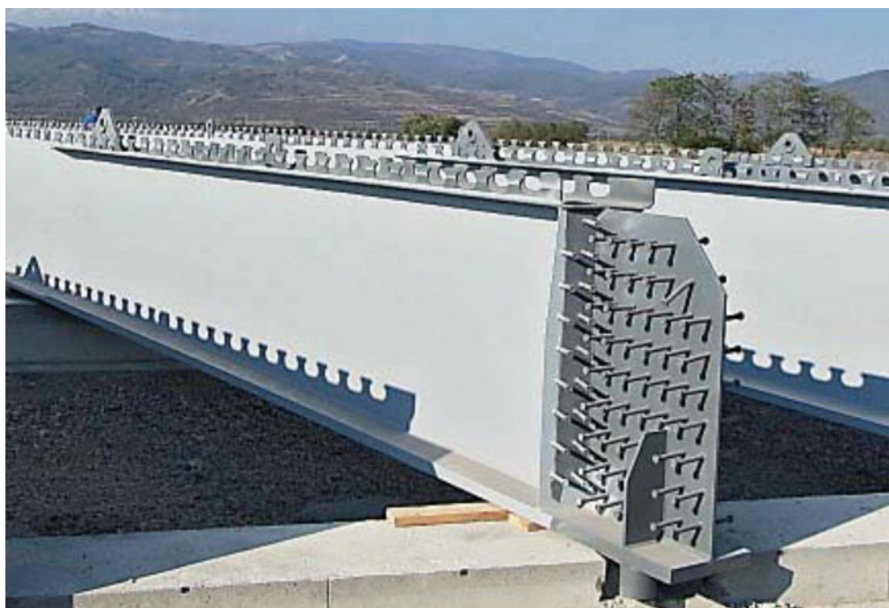
Figure 33: Figure 33 Steel girders on site
