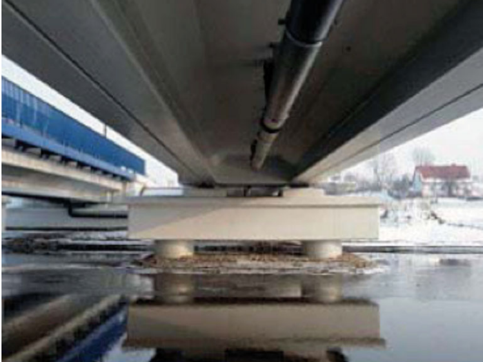
Figure 17: Bottom view on the railway bridge Łososina
