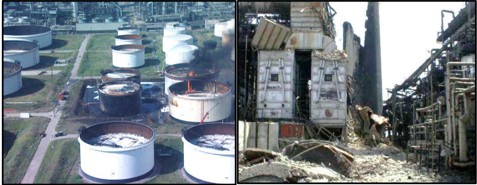
Figure 1: Damaged tanks at tank farm (left) and collapsed stack at TÜPRAŞ Refinery
