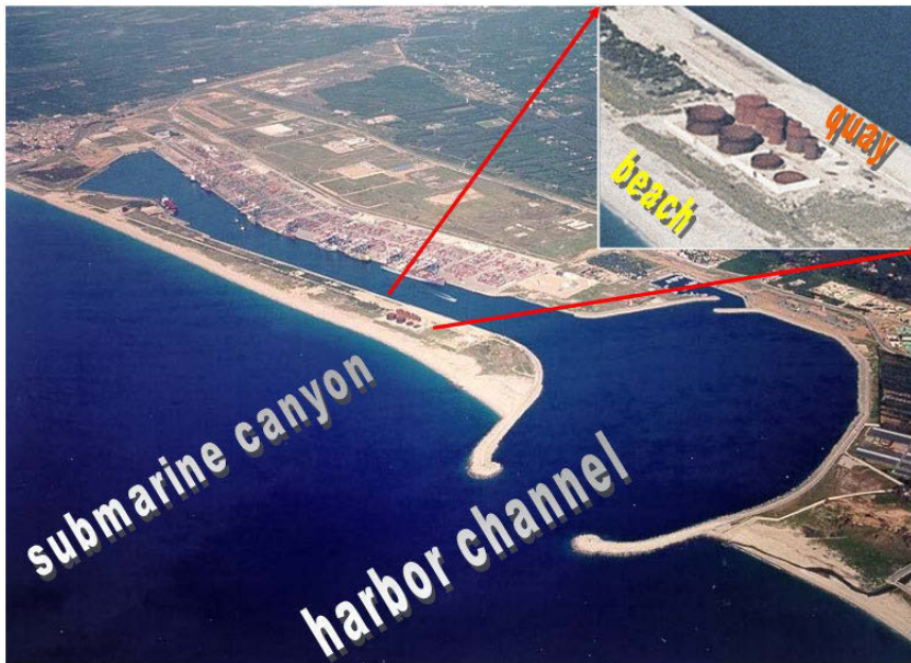
Figure 1: Aerial view of the critical facility
