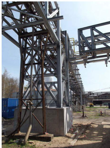
Figure 5: Replacement of a utilities bridge in full operation
