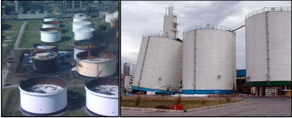
Figure 8: Damaged tanks at TUPRAS and insulated tanks at HABAŞ Facility
