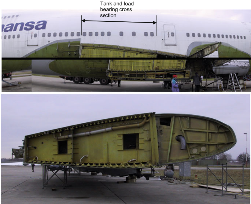
Fig. 14.14 View of the contact section of the wing to the fuselage; only the central third is designed as a load-bearing cross section and is simultaneously designed as a tank
