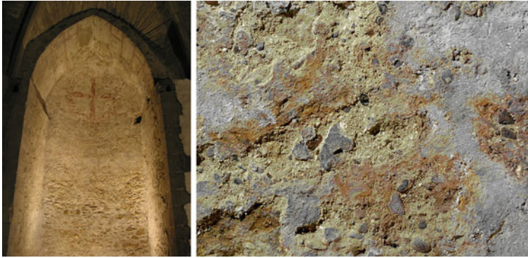
Fig. 4.32 St. Virgil's chapel (Vienna, Austria): halophilic bacteria and archaea cause a rosy stain on the salt-attacked stone surface of the Medieval monument
