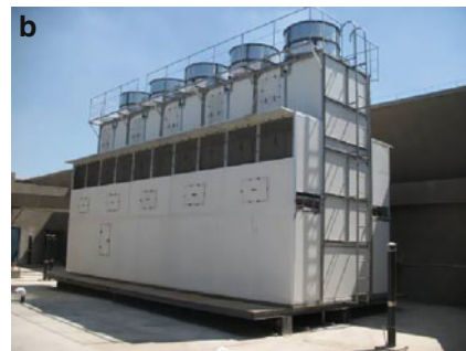
Fig. 8.18 Indirect evaporative chiller: (a) schematic and (b) photo
