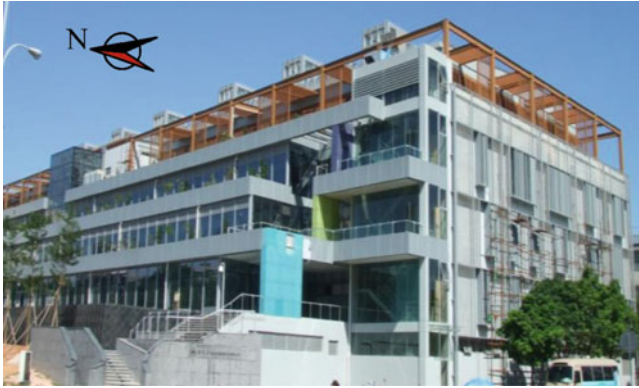
Fig. 8.1 The tested office building in Shenzhen
