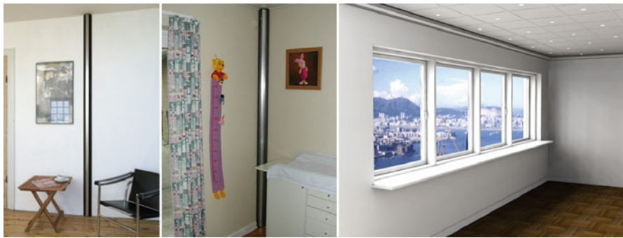
Fig. 3.32 Applications of the dry FCU units
