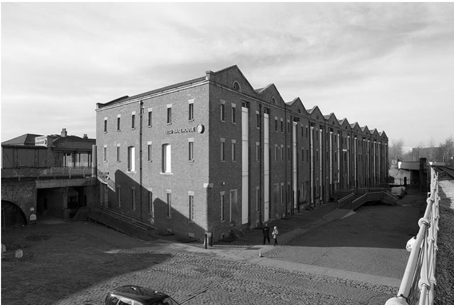
Fig. 1. The 1830 Warehouse (Image ©MOSI)
