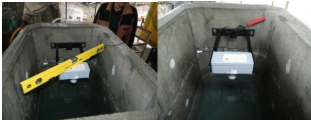
Fig. 11. Instrument installations, alignment and leveling and an Installed Unit
