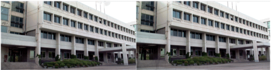
Fig. 1. CCTV video data through the building
