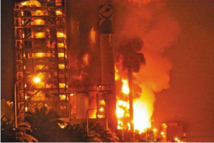
Fig. 1 A petroleum refinery plant fire accident
