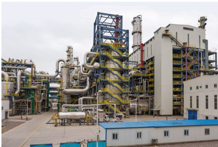
Fig. 6.84 Methanol-to-propylene plant at Shenhua Ningxia Coal Industry Site
