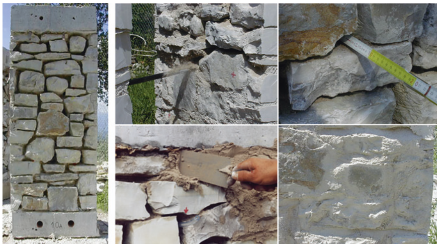
Fig. 9 Deep re-pointing procedure [7]
