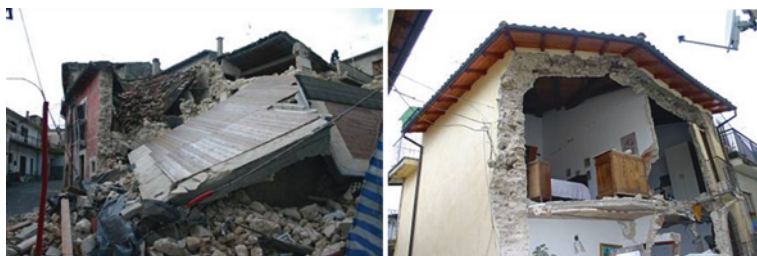
Fig. 7 Damage caused by past interventions, Abruzzo 2009
