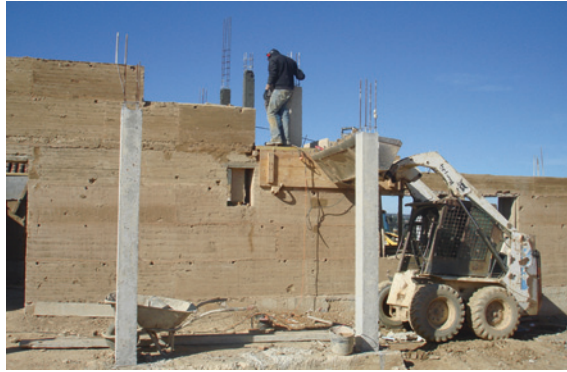
Fig. 1 Construction of a new rammed earth house in Odemira, Portugal
