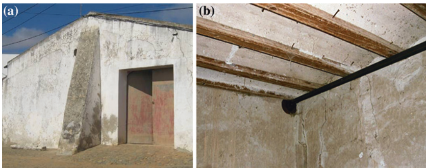
Fig. 8 Strengthening of rammed earth walls by means of: a buttressing [20]; b tie bars [5]
