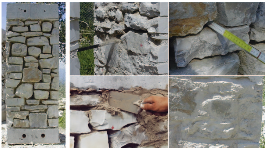
Fig. 9 Deep re-pointing procedure [7]
