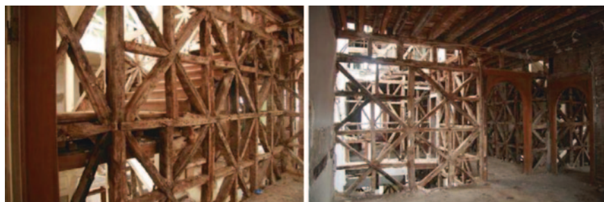
Fig. 1 Gaiola after removal of cover and masonry
