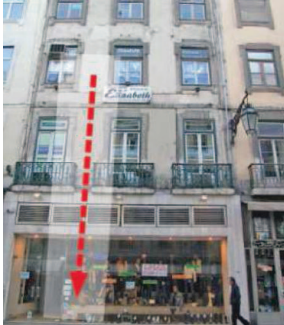
Fig. 22 Cut of columns at ground floor level [21]
