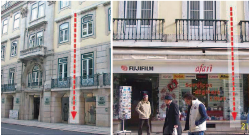
Fig. 43 External accesses and window shops with integration of original columns [21]
