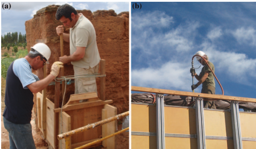
Fig. 3 Rammers used to compact rammed earth: a manual rammer; b pneumatic rammer (courtesy of Bly Windstorm from Earthdwell)
