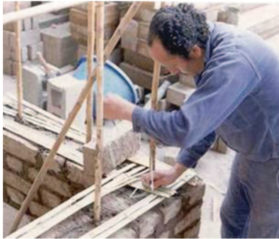
Fig. 27 Internal cane mesh reinforcement [77]
