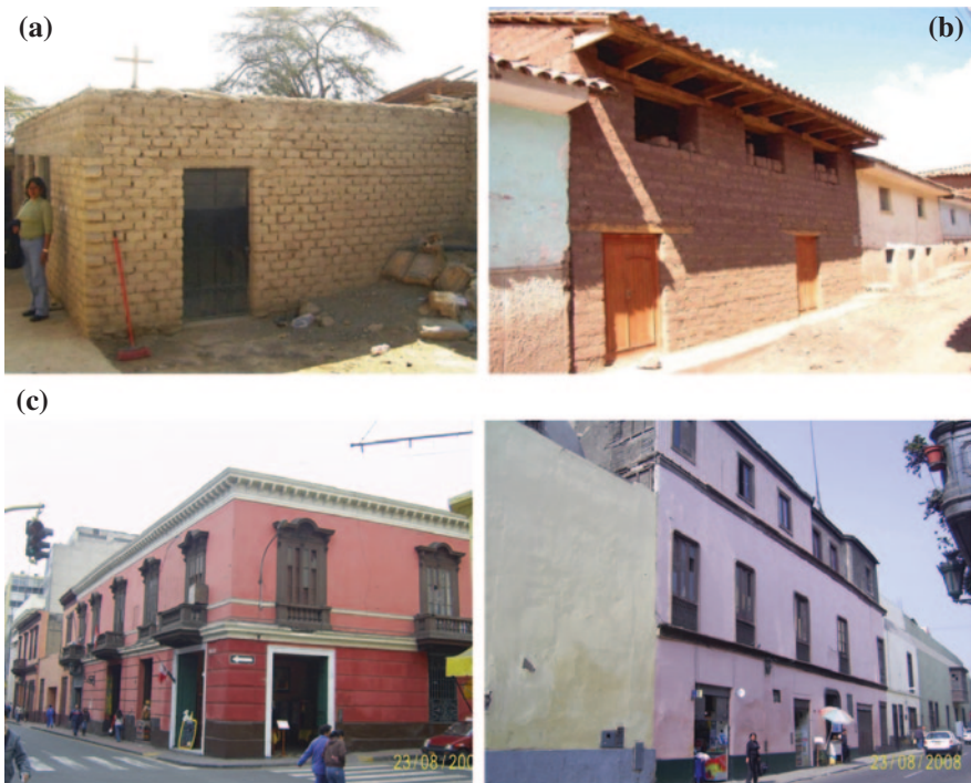
Fig. 4 Typical Peruvian adobe houses. a Adobe house located at the peruvian coast. b Adobe house in peruvian highland. c Colonial adobe houses of two and three storeys in Lima, Peru
