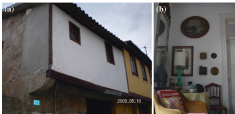
Fig. 14 Two examples of regularly maintained tabique buildings. a Example 1 ( exterior view ). b Example 2 ( interior view )
