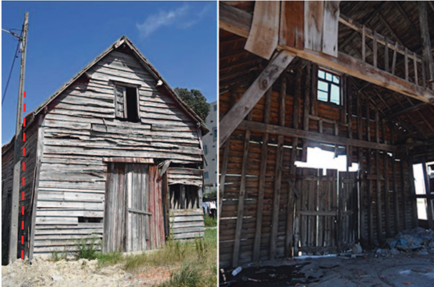
Fig. 13 Traditional timber constructions—Portugal (credit A. Tavares)
