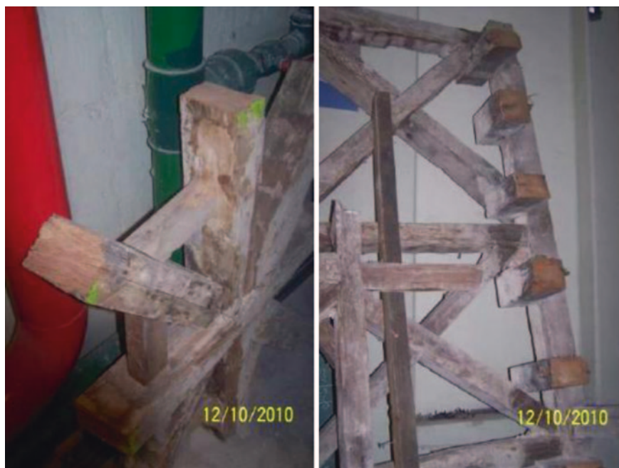
Fig. 19 Evidence of nowadays excellent conservation state of frontal walls
