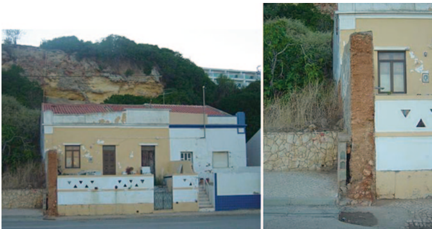
Fig. 7 Rammed earth construction, Portugal (credit H. Varum)
