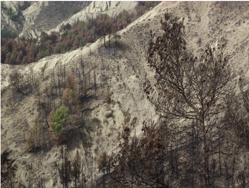
Fig. 4. Burnt area with surface instability phenomena
