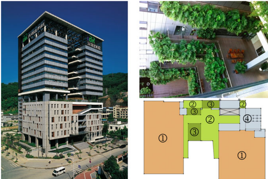
Fig. 43.1 Left: picture of the building’s southeast side. Top right: view on the central corridor platforms in the upper part of the building. Bottom right: schematic view of the floor plan of the upper part of the building; 1 (orange): working areas equipped with AC; 2 (light green): outside corridor and stairs; 3 (dark green): outside functional areas (for meeting, hot water, printers); 4 (gray): bathrooms, indoor stairs, elevators, and technical rooms
