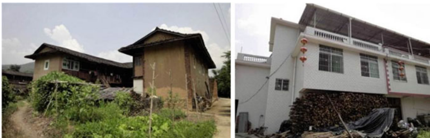
Fig. 41.2 The photograph of normal rural buildings built of rammed earth ( left ) and brick ( right )
