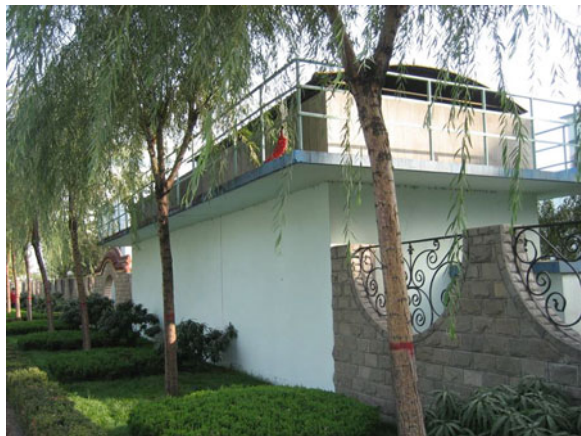
Fig. 66.1 Photograph of air shaft outlet of coal mine before reformation
