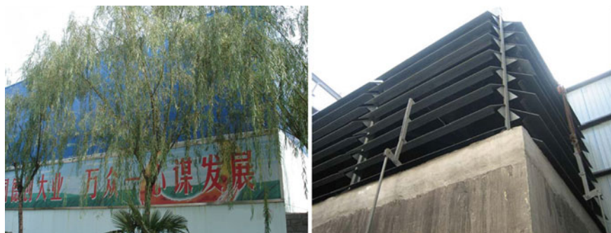
Fig. 66.15 The photograph of reformed fan diffuser in Xingdong Mine
