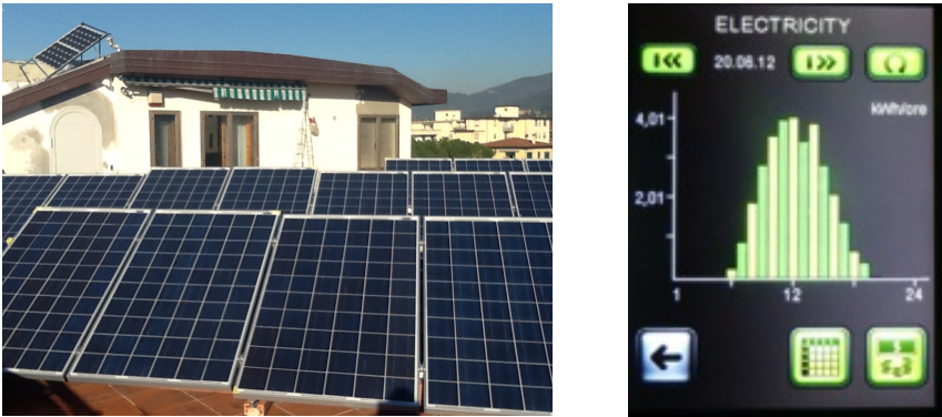
Fig. 3. Left: the terrace and roof are used for solar cell generation systems. Right: graph showing histogram of the generated energy in kWh during a sunny day on June 20, 2012.
