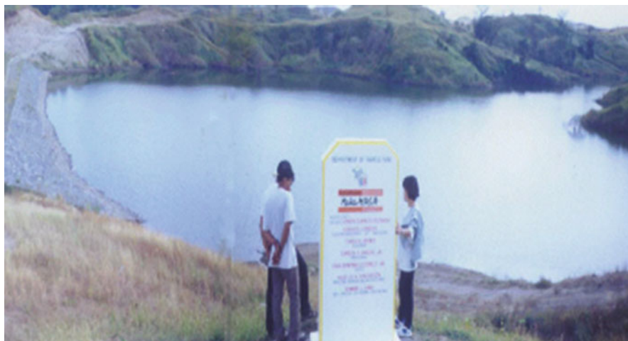
Fig. 2 Reservoir area of small water impounding project
