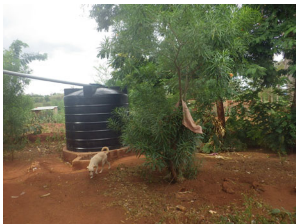
Fig. 1 Water tank 1 for domestic use
