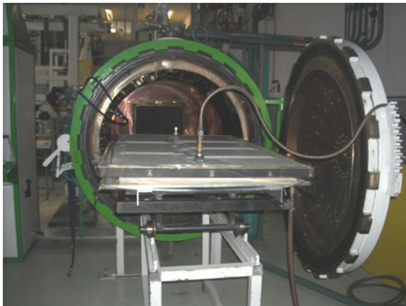
Fig. 1.4 Autoclave moulding (UPS, Toulouse)
