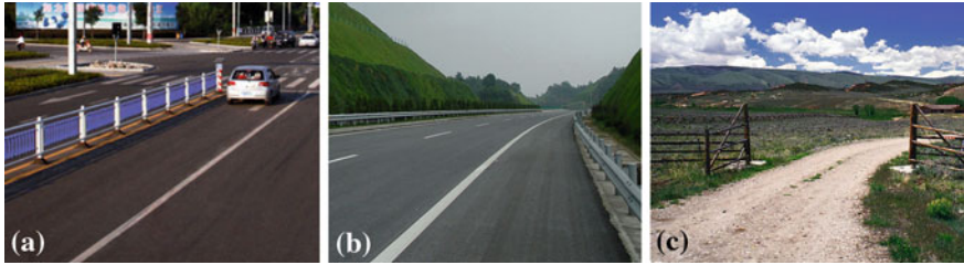
Fig. 1 The actual road. a Urban environment. b Highway. c Rural environment
