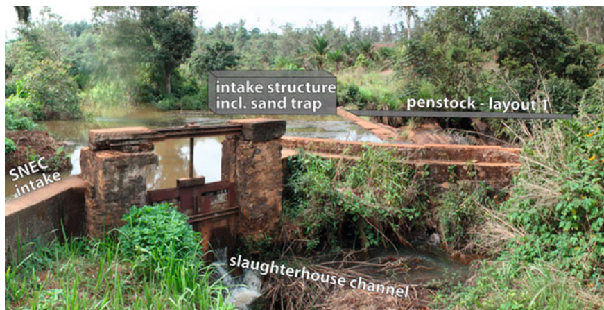
Fig. 12.9 Overview of intake situation at Cascade 1
