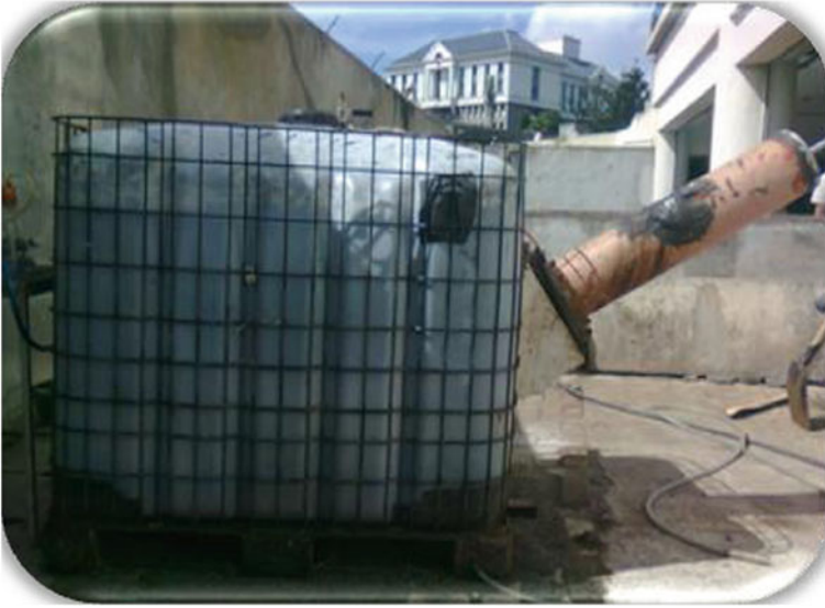
Fig. 37.3 Side view of digester
