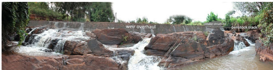
Fig. 12.1 Downstream view with weir overhaul and intake structure
