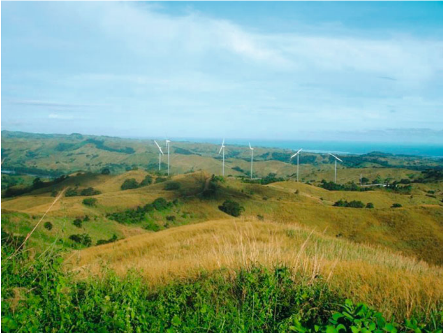
Fig. 1.1 Butoni wind farm in Fiji
