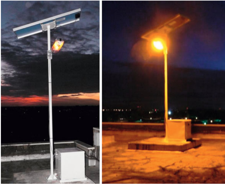
Fig. 26.6 PV-powered street lamp ( Photos courtesy of I. Haraksingh )
