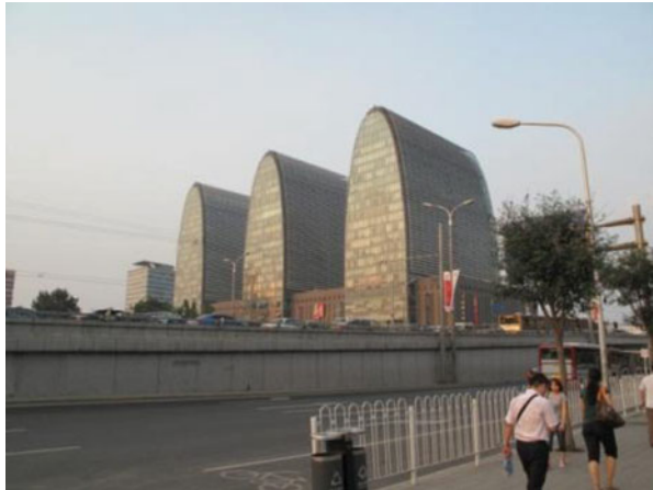
Fig. 29.4 The aerial view of Cade Mall
