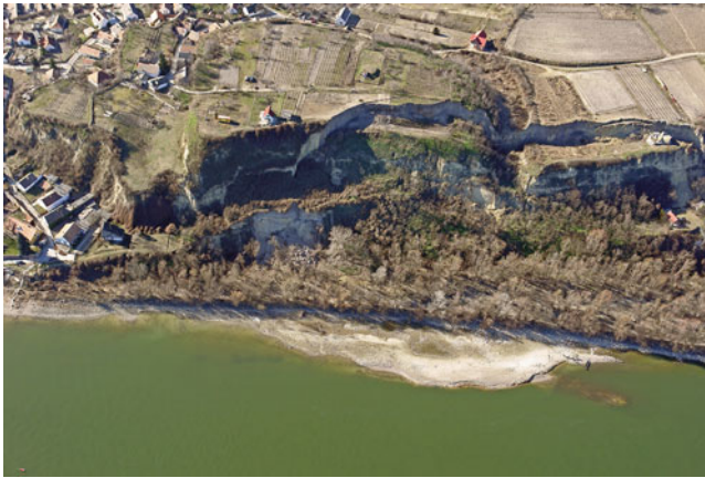
Fig. 1 Oblique aerial view of the Dunaszekcső landslide. Photo was taken by László Körmeny on February 17, 2008
