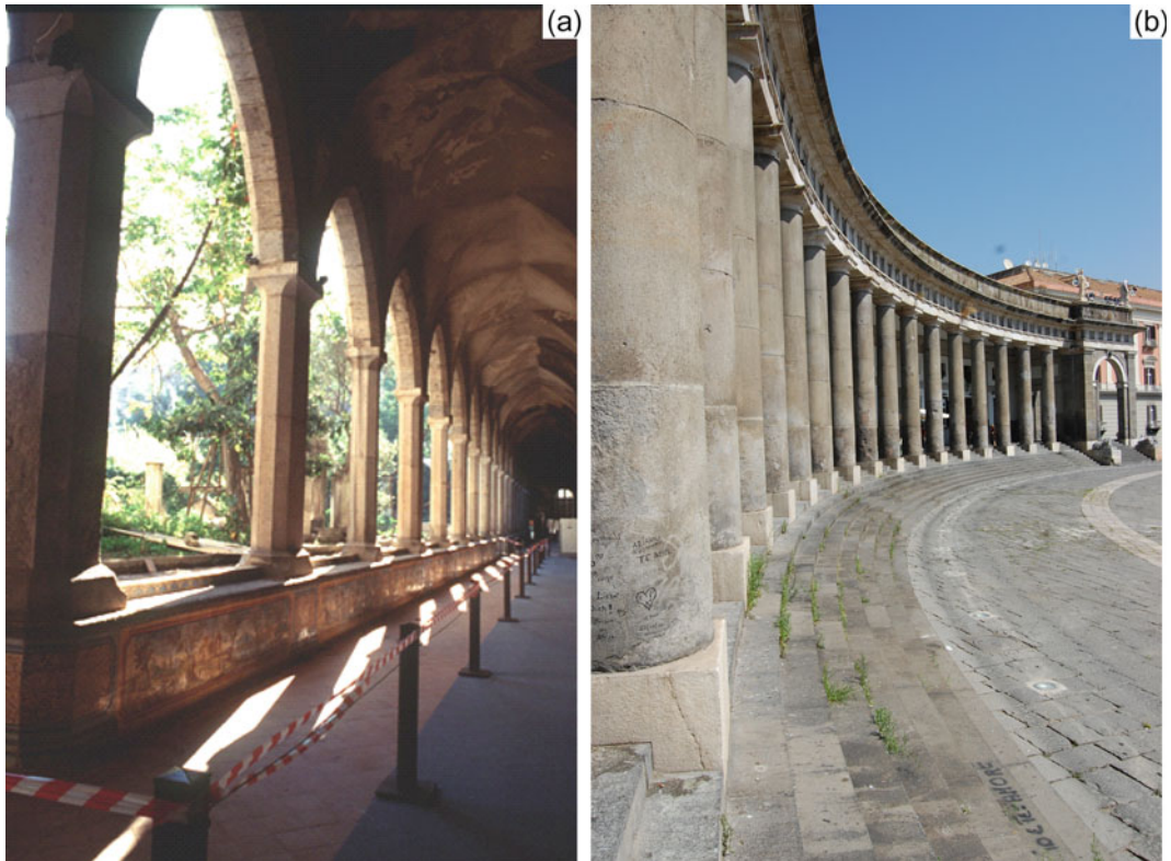
Fig. 9 The Phlegraean trachytic lava in the monumental architecture of Naples. a Colonnade of the Santa Chiara Monastery cloister (photo by M. d'Albora); b colonnade of San Francesco di Paola Church. (photo by A. Langella)
