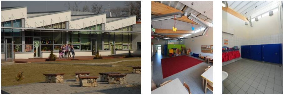
Fig. 6. In the preschool area there is a shed roof allowing direct eastern daylight into the rooms and also into half of toilets. a) the shed roof from outside, b) the natural light penetrating the classrooms, c) the restroom illuminated by natural light
