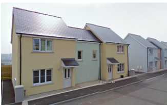
Fig. 1. Britannia Drive south elevation as-built, before installation of photovoltaic panels
