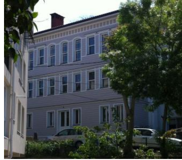
Fig. 2. The reconstructed building according to the old legislation
