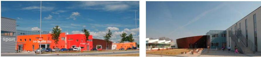
Fig. 1. a) View towards school entrance zone with distinct volumes housing different functions. b) View towards a courtyard between school and preschool wing. A copper volume with dining room is shared by the two functions.
