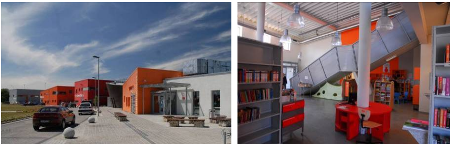
Fig. 4. Distinct volumes with separate entrances for different functions shared with local community a) View towards entrance area, b) School and community shared library
