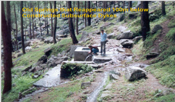
Revival of old spring below constructed subsurface dykes
