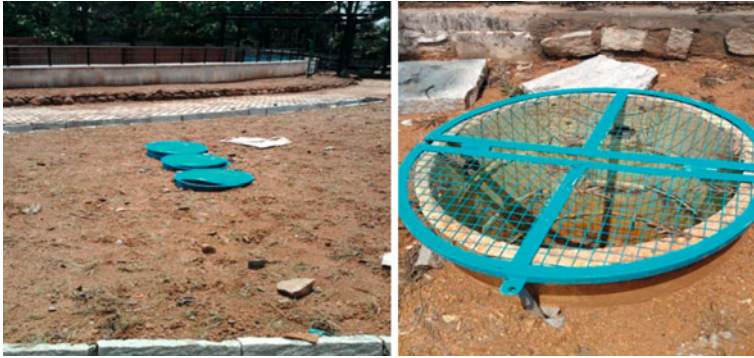
Plate 2 Model of Ground water recharge pit, RWH Theme Park, Photo Manasi S
