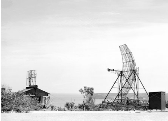
Fig. 5.2 LW/AWH (Light Weight Aircraft Warning, Height) prototype 25 cm radar with size of antenna 25 by 12 ft. (7.6 by 3.6 m), located at Georges Heights, Middle Harbour, Sydney (note South Head in the distance). The magnetrons were designed at the University of Melbourne and manufactured by AWA. Pulse lengths were either 4 or 1 \mu s, with a power of 500 kW. Weight was only 7 t compared to 35 t for comparable UK and US radars. This radar was the major technological achievement of RPL during World War II. The end of the war brought a cessation to development activities; only a few prototypes were built. The other antenna to the left is the communications aerial for control of the radar. This radar spearheaded RPL's post-war drive to solve civilian problems for control of aircraft traffic (CSIRO Radio Astronomy Image Archive B1362)
