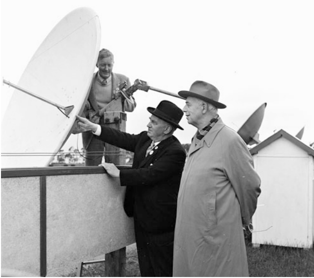
Fig. 11.5 URSI tour of Potts Hill Reservoir Field Station, August 1952. Here Chris Christiansen ( left ) describes the new 32-element east-west grating array, opened November 1951. Sir Edward Appleton, President of URSI, points to one of the 1.7 m antennas. To the extreme right is Prof. Balthasar van der Pol, Director of CCIR in Geneva and prominent Dutch radiophysicist. Note the URSI pin on the jackets of Appleton and Christiansen (Fig. 11.2) (CSIRO Radio Astronomy Image Archive B2842-R6)
