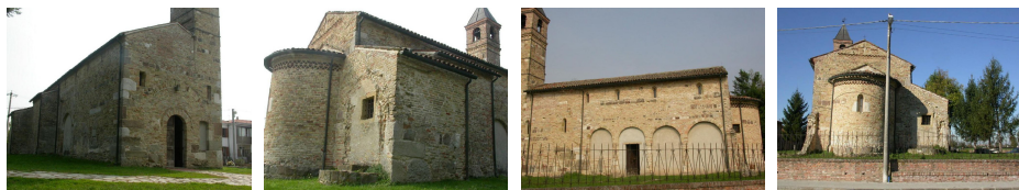
Fig. 9. Canonical views for the pozzoveggiani data set. One image was selected for each side of the church.
