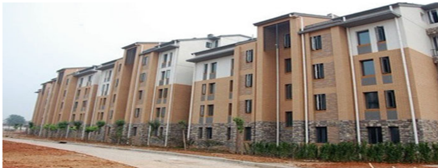
Fig. 110.1 Dwelling construction where the quantification model is applied in the case study
