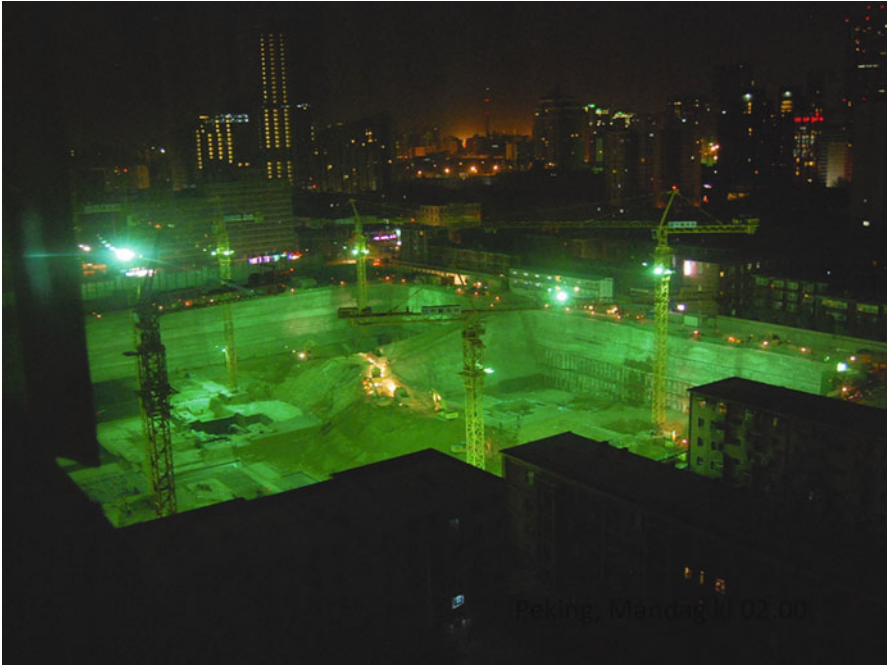
Fig. 66.4 Five excavators working during night at a construction site in Beijing
